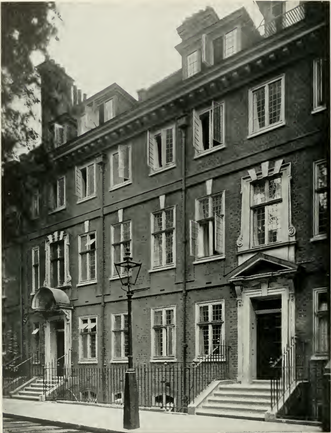
TWO URBAN HOUSES, 14 AND 15, GREAT COLLEGE STREET, WESTMINSTER, LONDON: BUILT ON THE SITE OF TWO OLD HOUSES WHICH WERE CONDEMNED. THEY ARE FACED EXTERNALLY WITH LIGHT RED DRESSINGS AND DARKER BRICKS FOR FILLING. THE ENTRANCE DOORS HAVE STONE DRESSINGS
